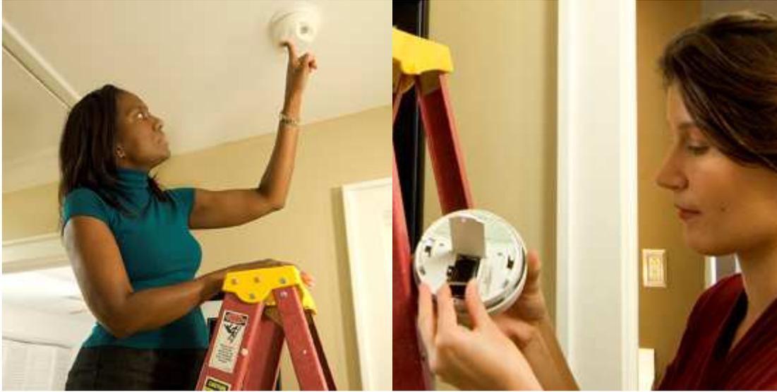
Is your smoke alarm still working? Smoke alarms *must* be maintained! A smoke alarm with a dead or missing battery is the same as having no smoke alarm at all.
